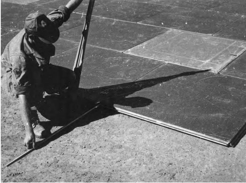
A soldier of the 20th Engineer Battalion places MX19 matting at New Plei Djereng Special Forces camp.
